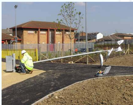
Left & above: Marlec's purpose designed raise and lower column makes installation and maintenance safe at ground level and avoids the cost of platforms
