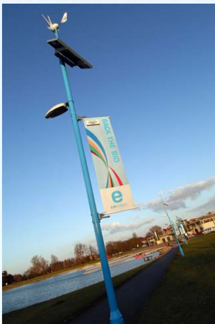
One of 5 Green Columns installed at the Olympic bid site in 2005.
